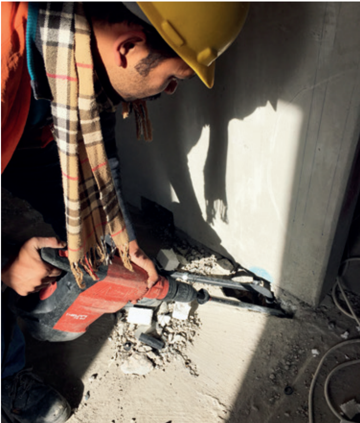
The Hilti combihammer TE 60 is the perfect allrounder for drilling (15-40 mm) and medium-duty chiseling in concrete.
