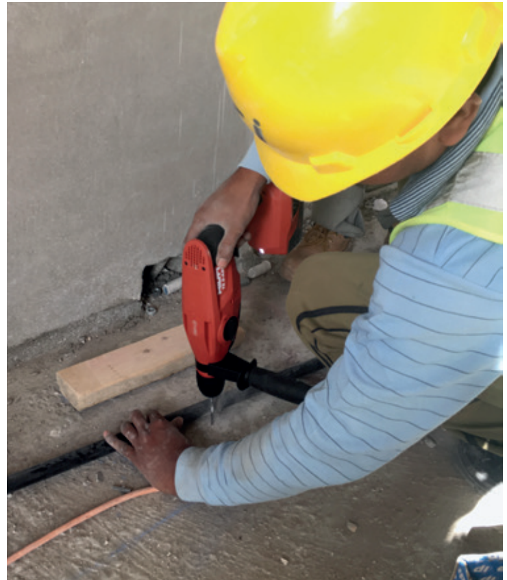
The Hilti cordless rotary hammer TE 2-A22 is a powerful drilling tool (4-16 mm) for light duty drilling in concrete and masonry.
