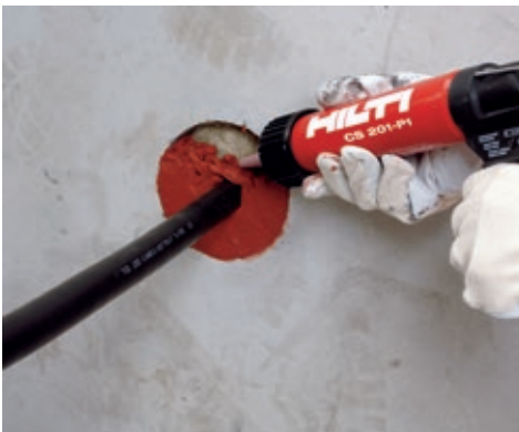
FS-ONE MAX can be used for closed or vented plastic pipes.
