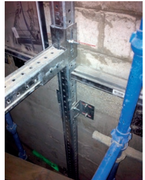
MQ Systems are been used for the divider beam.
