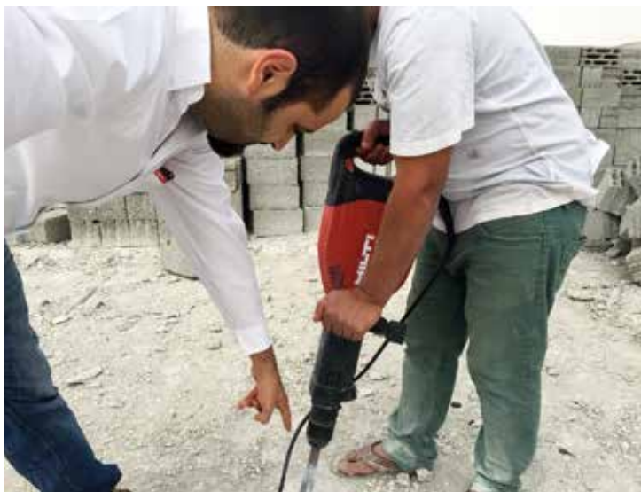
Working on site with the Hilti breaker TE 1500 saves time and efforts compared to air systems.
