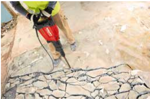
Demolishing concrete and masonry at floor level or below waist level.
