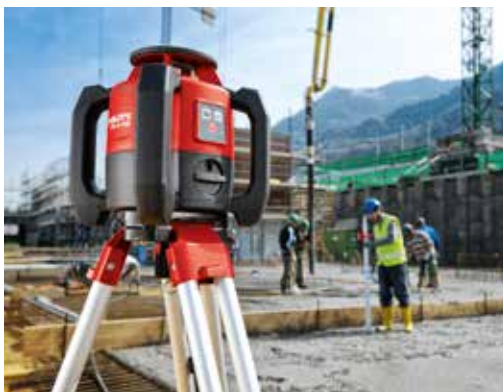
Checking levels when pouring concrete.
