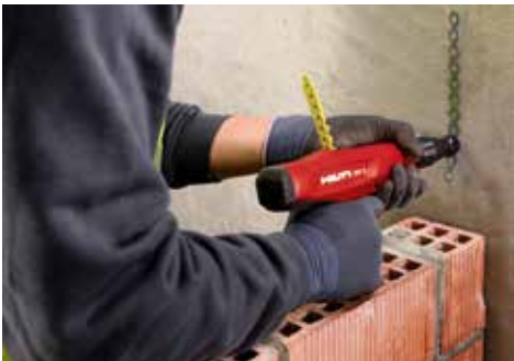
Fastening wall tie to concrete.
