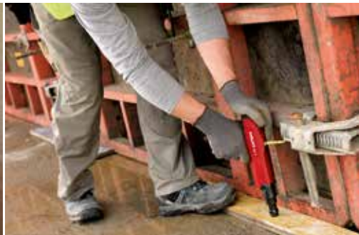
Fastening wood to concrete (e.g. formwork).
