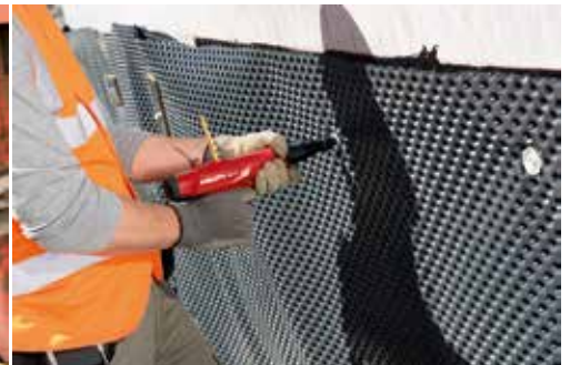
Fixing membrane to concrete
