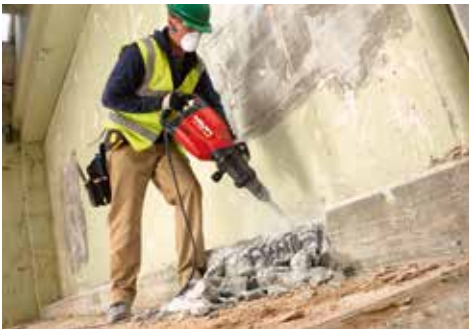
Corrective chiseling such as adjustments to door and window openings.
