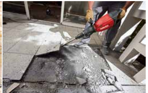
Removing tiles, bushing and compacting.
