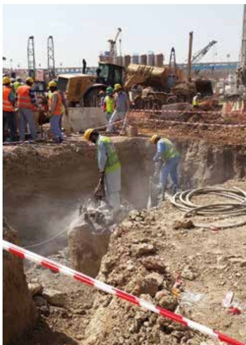
Hilti TE 3000 competing with an air compressor breaker. The electric system is clearly more convenient.
