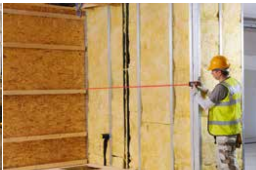
Positioning drywall quickly and accurately.
