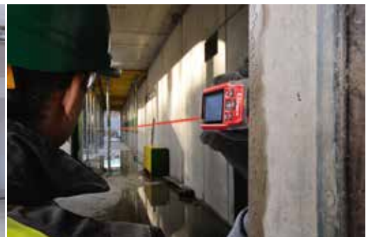
Measuring lengths, heights and widths for different construction applications.
