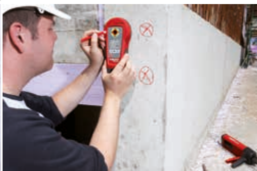
The Hilti PS 35 finds the position and depth of reinforcing bars for an efficient anchor fastening.
