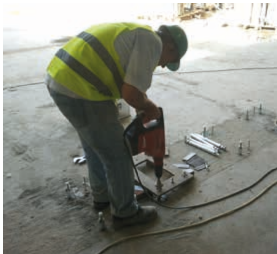
To apply the right expansion to the HDA anchor Orascom uses the Hilti combihammer TE 70.
