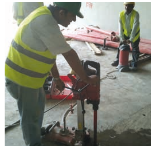
Orascom used Hilti diamond coring for drilling the anchor holes through rebar, without producing any concrete cracks.
