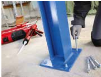
2 Structural steel connections to concrete
